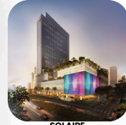
SOLAIRE QUEZON CITY
